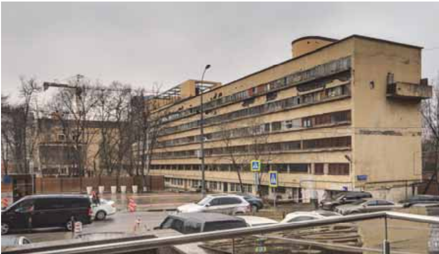
Fig. 4. Dom-kommuna of Narkomfin. Arch. Moisey Ginzburg, Ignaty Milinis, 1928–30. Photo from 2017.
