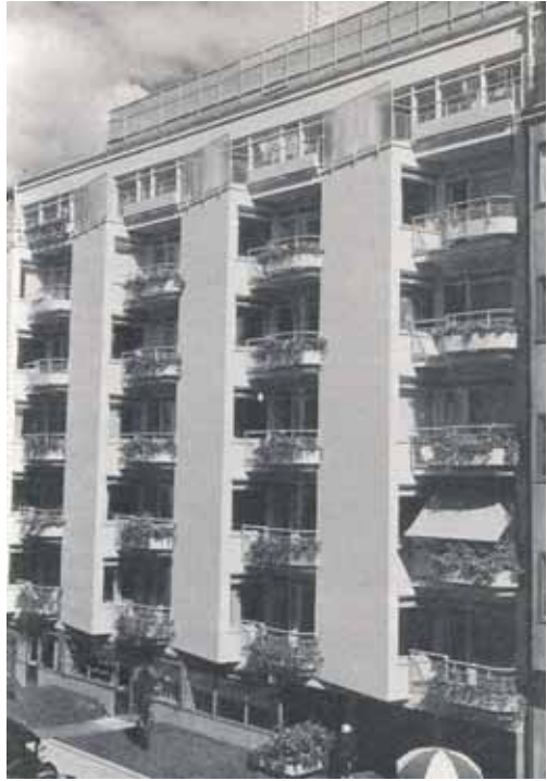
Fig. 7. Collective House on John Ericssonsgatan 6. Arch. Sven Markelius, 1934. Photo from 1936.
