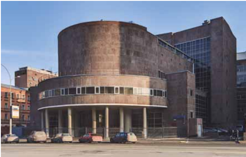
Fig. 3. The Tsentrosoyuz Building in Moscow. Arch. Le Corbusier and Paul Jeanneret, 1928–30
