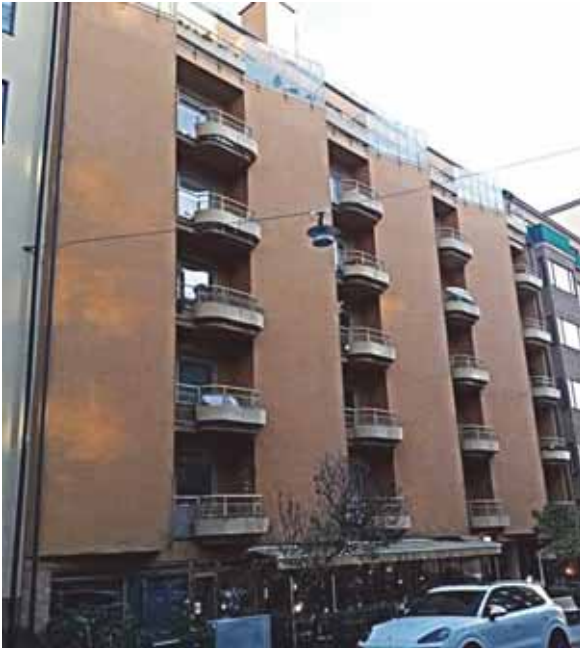
Fig. 6. Collective House on John Ericssonsgatan 6. Arch. Sven Markelius, 1934. Photo from 2018.
